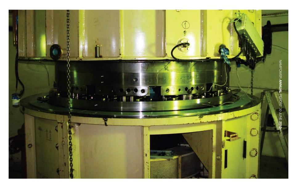
Ruacana turbine view of main shaft, thrust and turbine guide bearing
