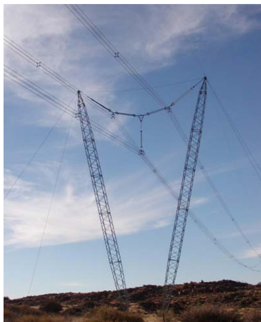
Figure 3-5: Compact Cross Rope Suspension Tower
