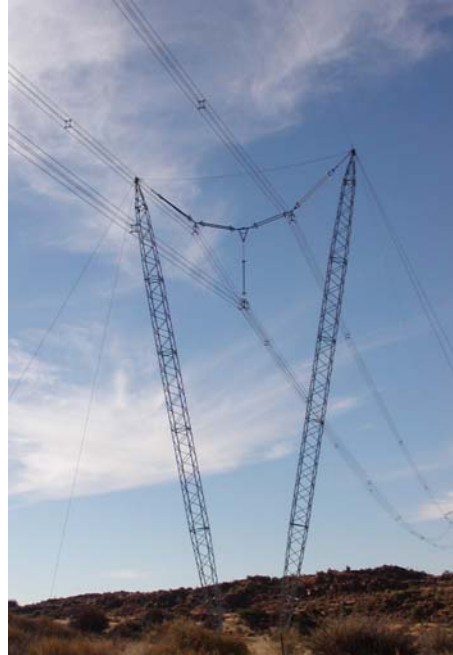
Figure 2: Cross-roped suspension tower
