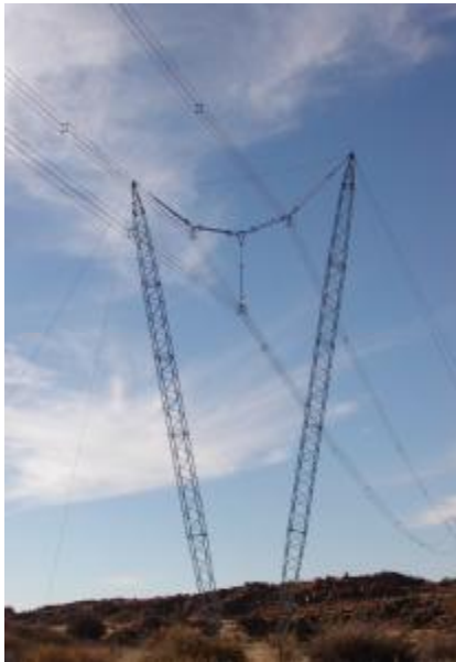
Figure 2: The structure of the proposed 220 kV line
