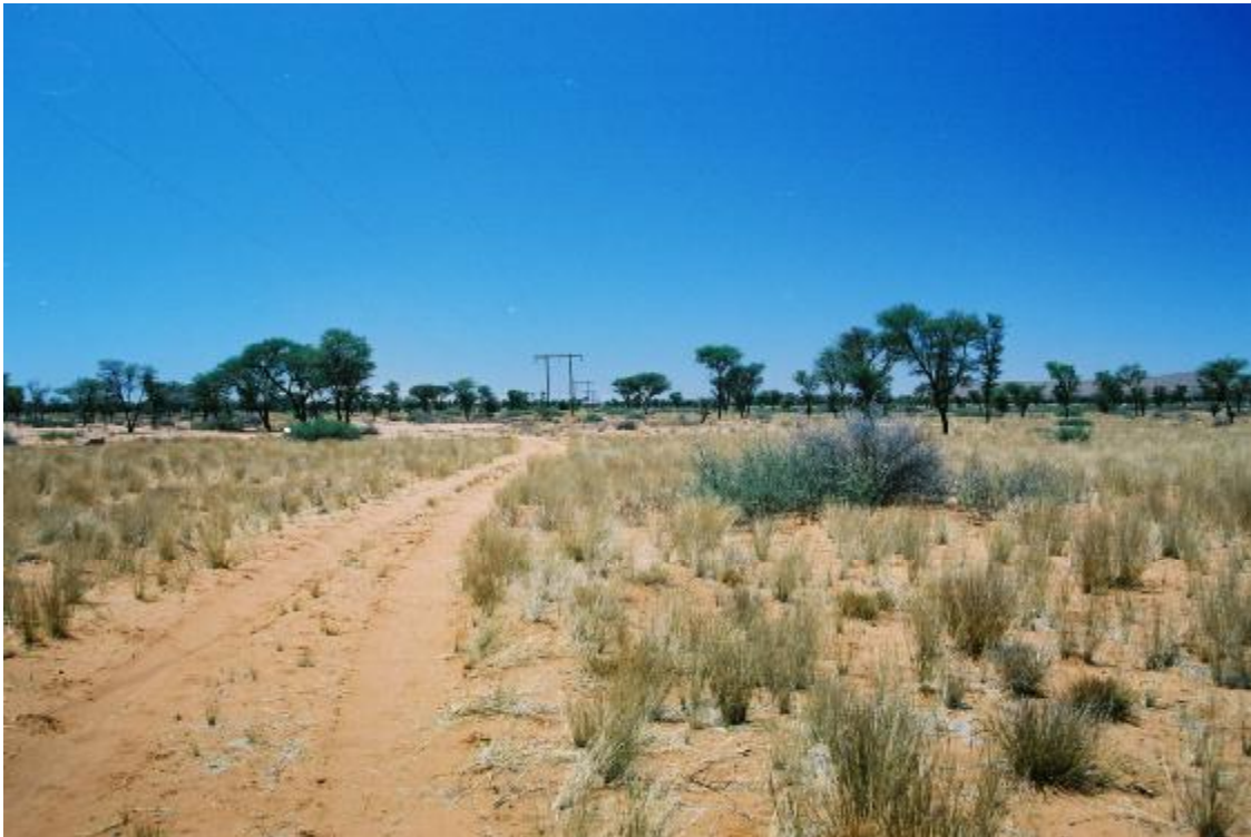
Figure 15: The servitude along the existing 66 kV distribution line to the east could be widened to accommodate the new power line. A service road already exists here.
