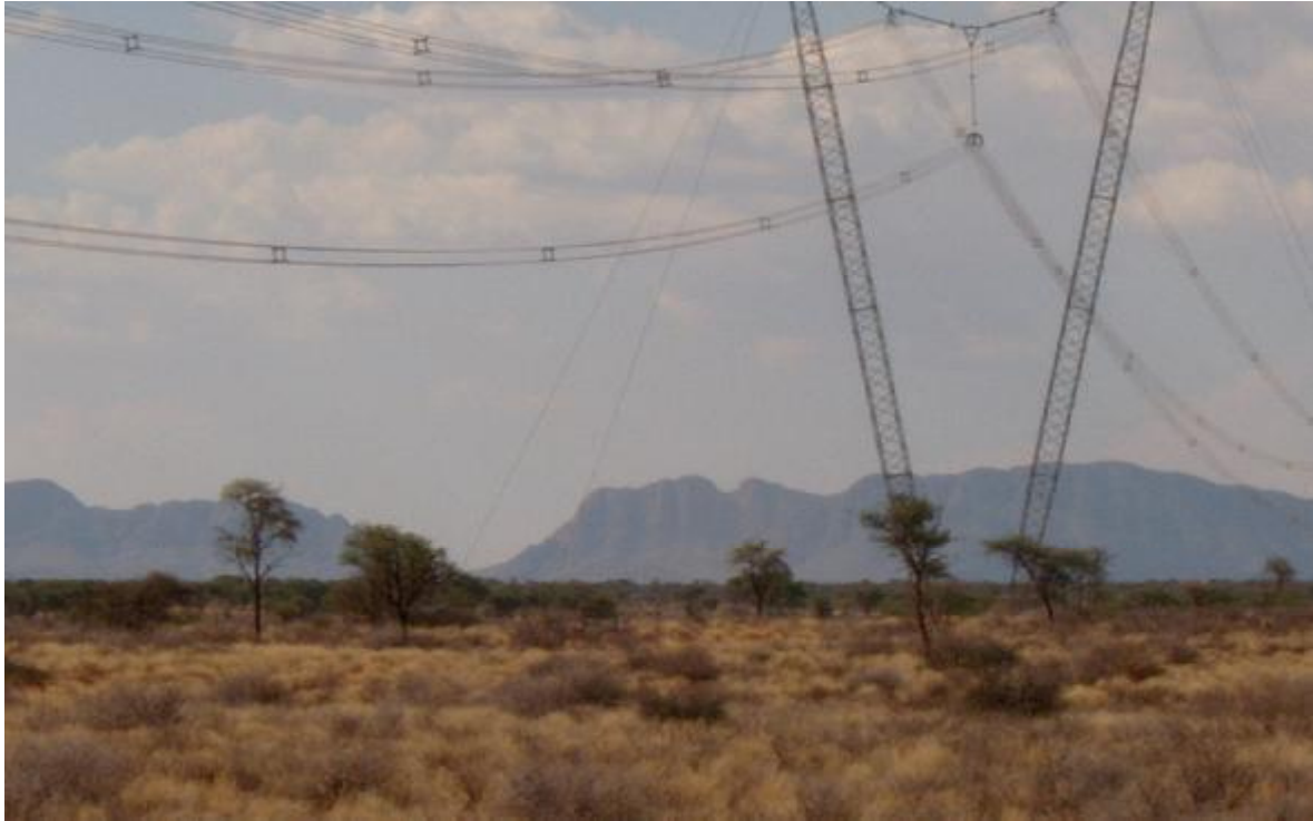
Figure 4: Photographic evidence - visual impact and electrocutions
