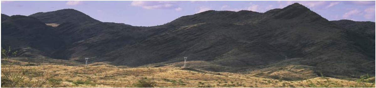
Photo 30: Where the sun can highlight the towers against a dark hillside, the powerline can have its greatest visual impact. These situations should be avoided if at all possible.
