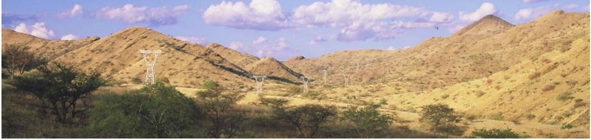
Photo 29: A new powerline in sunlight against a sunlit hillside is conspicuous. Reducing the reflectivity of the towers eg by painting or oiling them may reduce the visual impact to a minor degree.
