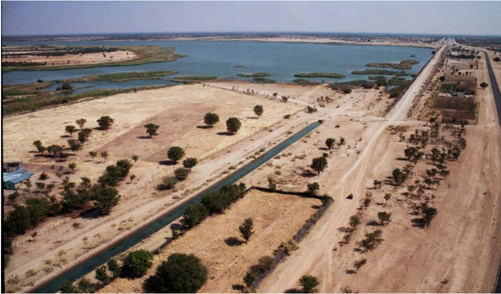
Photo 27: Onesi Dam on the south side of the tar road (C46). The width of the dam on the south side of the road is an obstacle for the powerline, which will therefore follow the road on its north side (out of this photo) where the dam is much narrower. Immediately west of the dam the preferred route crosses to the south side of the road again. The areas near the road are highly disturbed even though the density of settlement is low.
