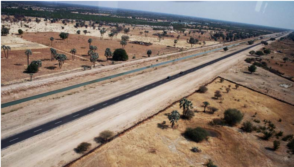
Photo 25: West of point O, the preferred route crosses to the north side of the tar road (C46) to Ruacana, which is shown running parallel with the canal. Note the large fruit trees and palms that will need to be avoided as far as possible.
