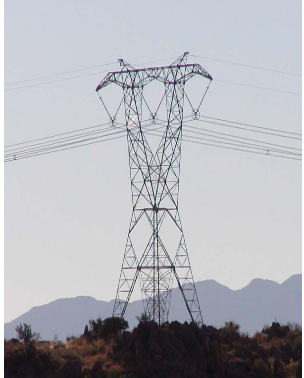
Photo 2: Self-supporting towers: four-legged structures with cables suspended. Strain-towers are similar but the conductors are attached directly to the cross arm.
