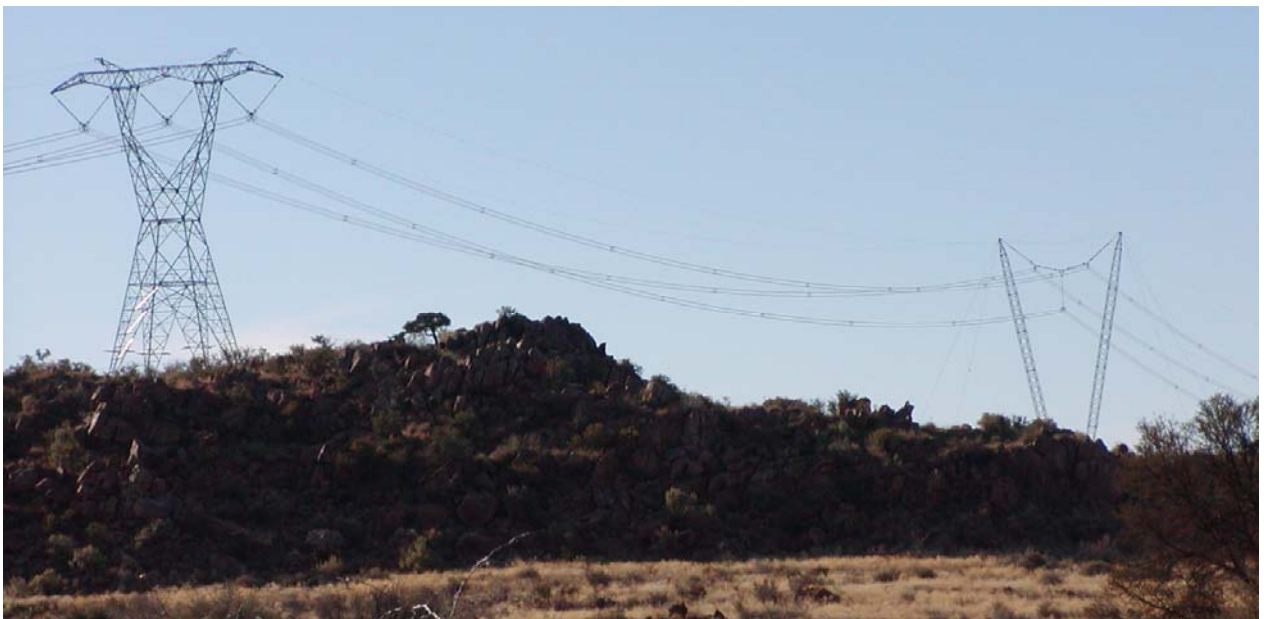
Photo 3: Self-supporting tower and Cross rope suspension towers in combination
