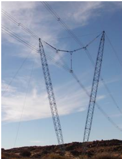
Figure 2 – Cross Rope Suspension Tower
